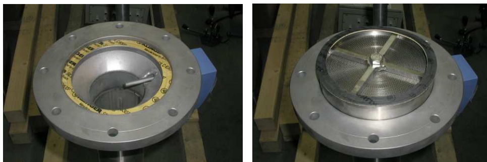
Fig. 6. Installation des joints
